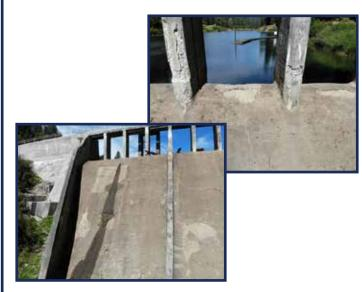
however, consists mainly of concrete with very few moving parts that wear out. Other than small concrete patching projects, the dam has operated for several decades without requiring a major maintenance project. However, in the last five years the concrete on the surface of the dam has deteriorated significantly and requires rehabilitation.
