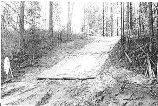
Installation of Erosion Mat on Slope above 16 inch Water Main
