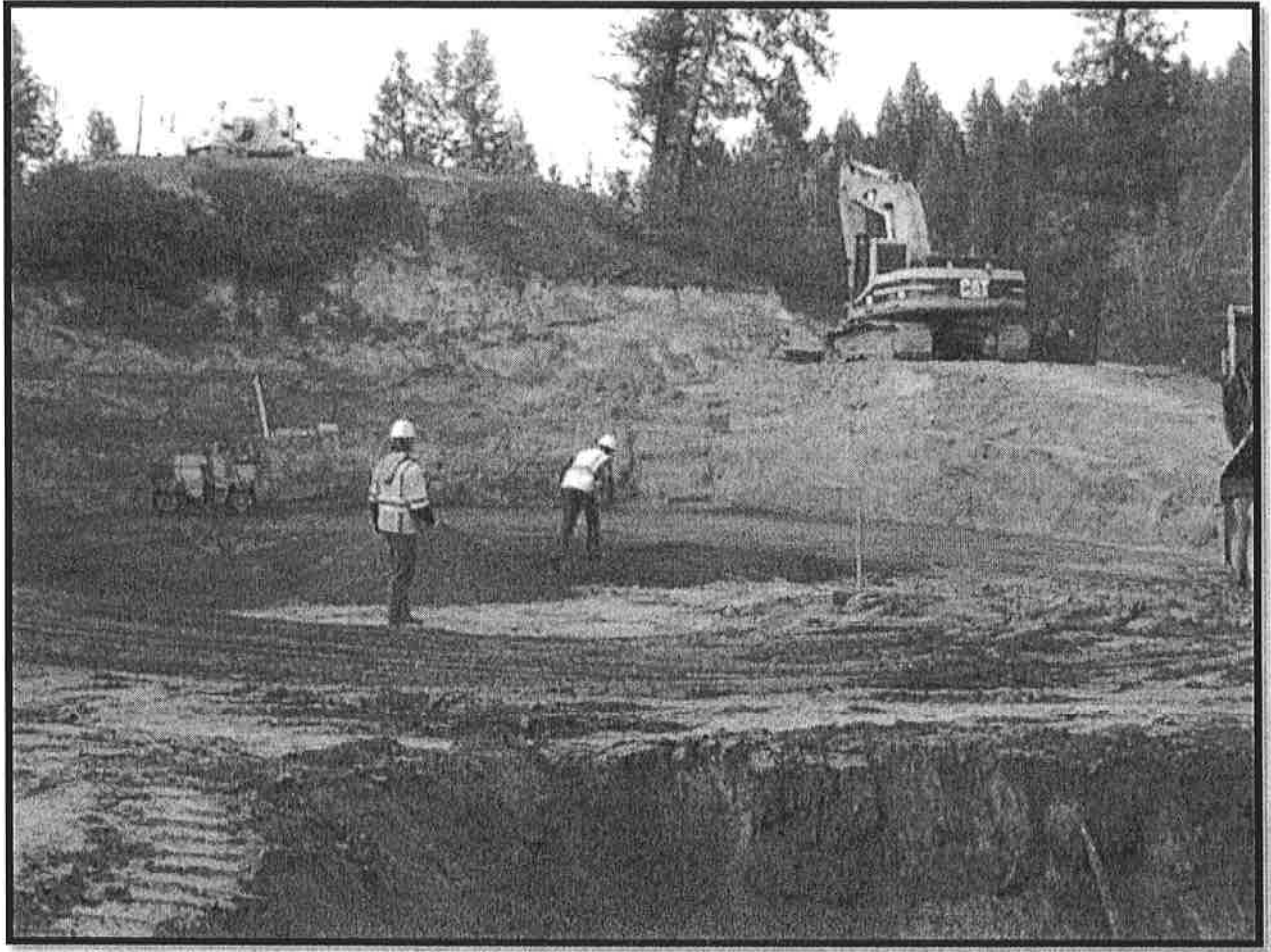
Prep tank base 11.10.11
