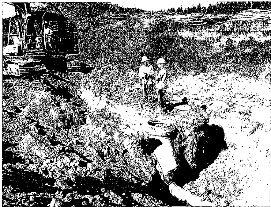
Crews work to relocate a water main along Highway 95 in conjunction with Idaho Transportation Department.
