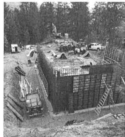
Forming walls-north half
