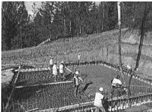
Pouring slab-north half
