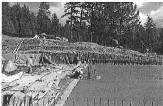
Finish work-south slab
