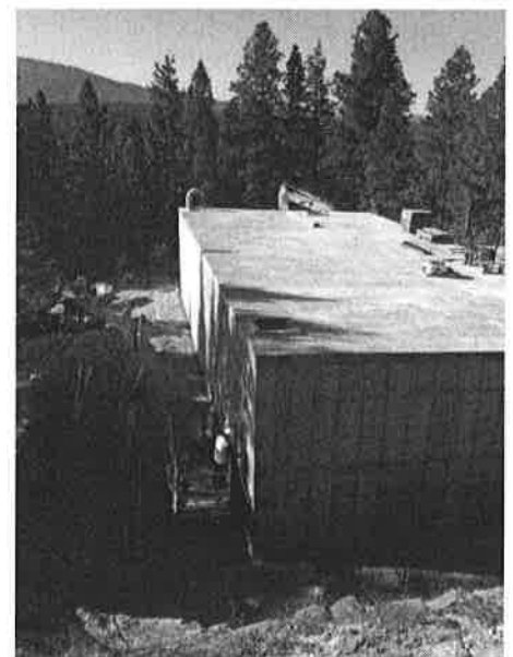
New Structure-Looking South
