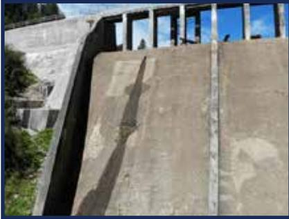
however, consists mainly of concrete with very few moving parts that wear out. Other than small concrete patching projects, the dam has operated for several decades without requiring a major maintenance project. However, in the last five years the concrete on the surface of the dam has deteriorated significantly and requires rehabilitation.
