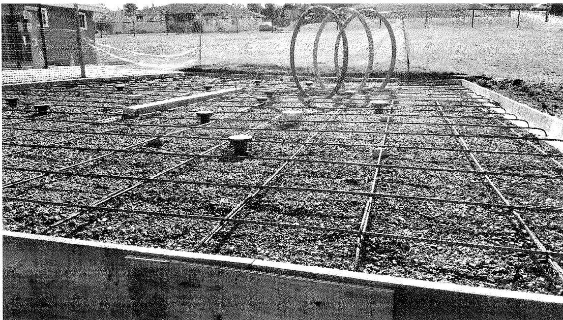
Photo of rebar and risers for splash pad features (June 23, 2020)
