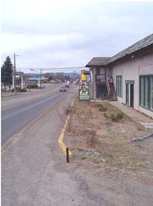
Travelers are the Key Market for South Hill Businesses. Uninviting to drivers and dangerous to pedestrians, much of South Hill's highway corridor needs substantial redesign
