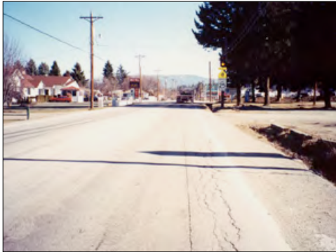
Deteriorated pavement and open drainage ditch on U.S. 95 at South Hill.
