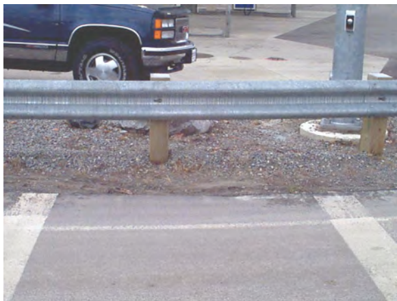
Absence of turn lanes and pedestrian safety measures are two of South Hill's biggest challenges. Note that the crosswalk (lower photo) actually is blocked by a highway guard rail!
