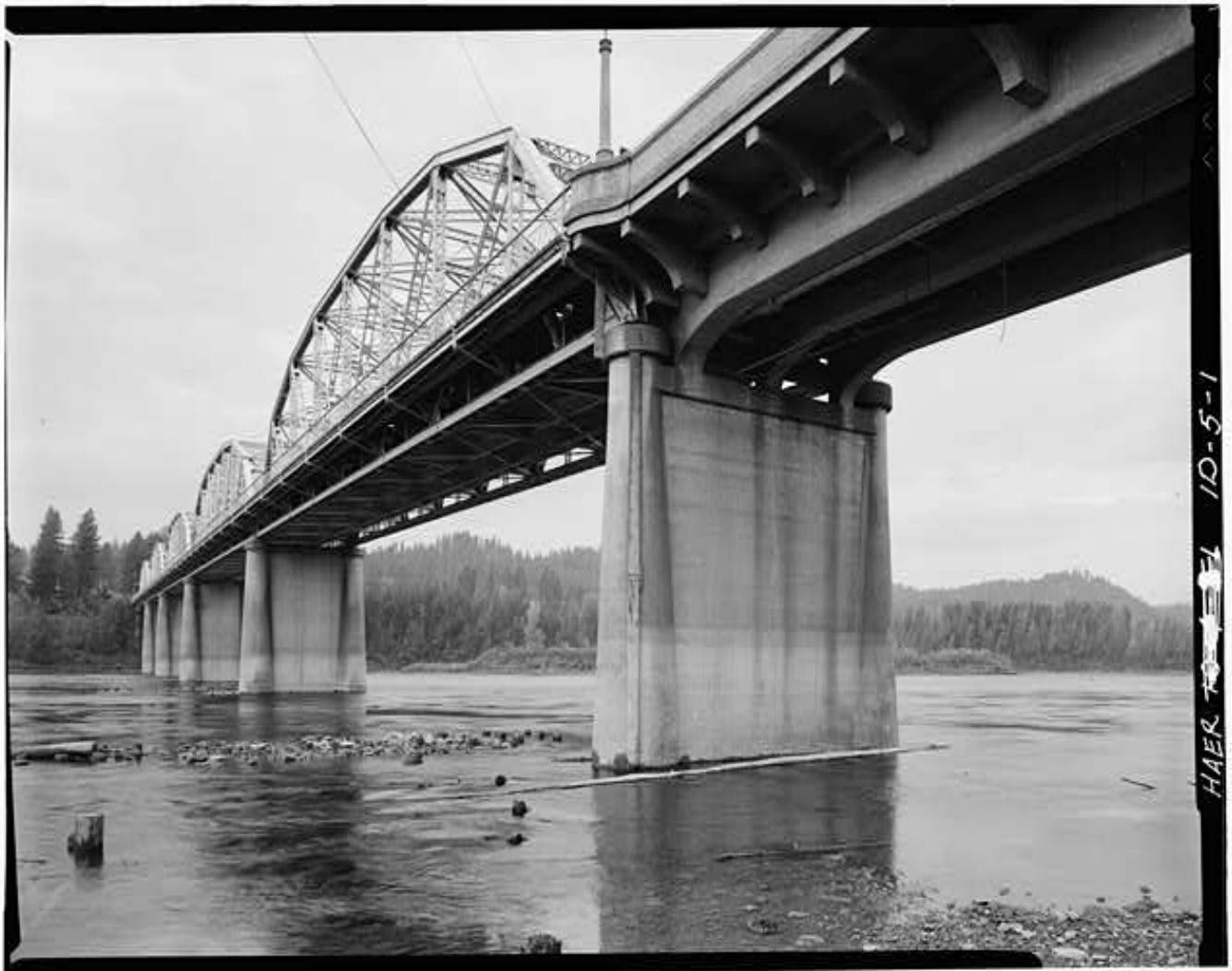
Bonners Ferry Bridge, Spanning Kootenai River, Photo Source: Library of Congress Prints and Photographs Division
