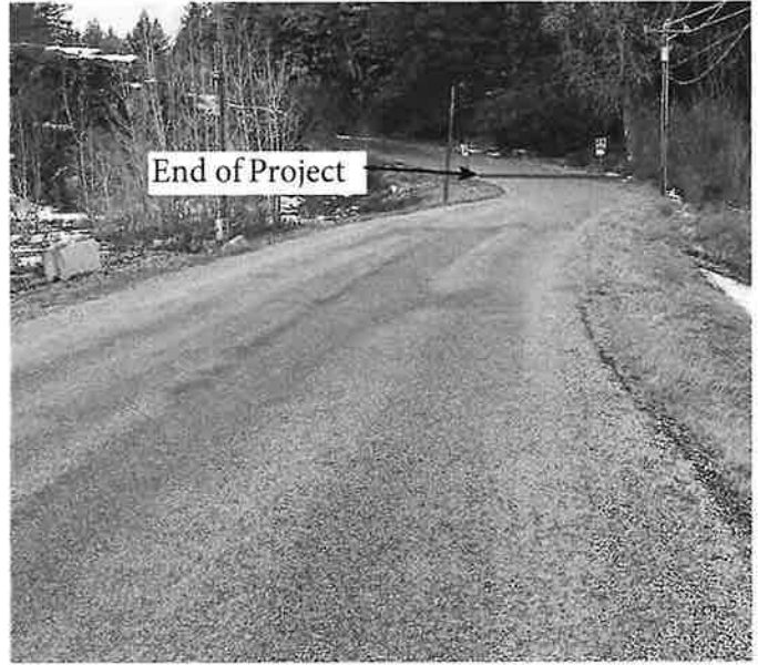
(6) End of project, facing west.
