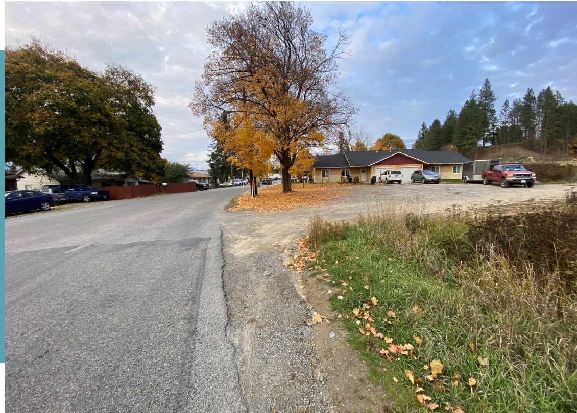
Photo 1: At Alderson, looking north at new street
