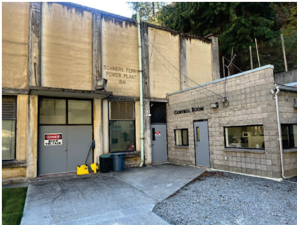
Figure 4.3-5. Powerhouse No. 2 (left) and control room (right).
