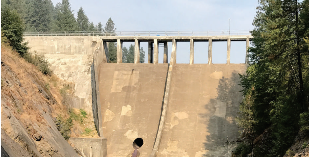
Figure 4.3-3. Moyie Dam spillway and low-level outlet.
