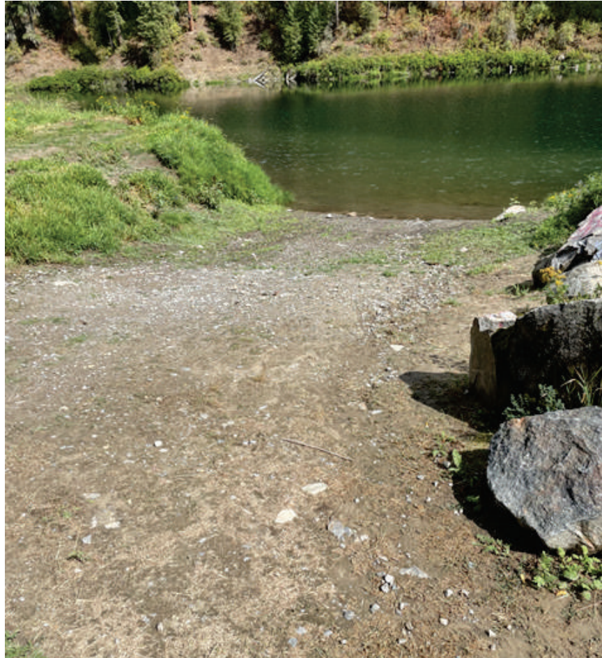
Figure 4.3-6. Project boating take-out and day-use area—gravel surface boat ramp.
