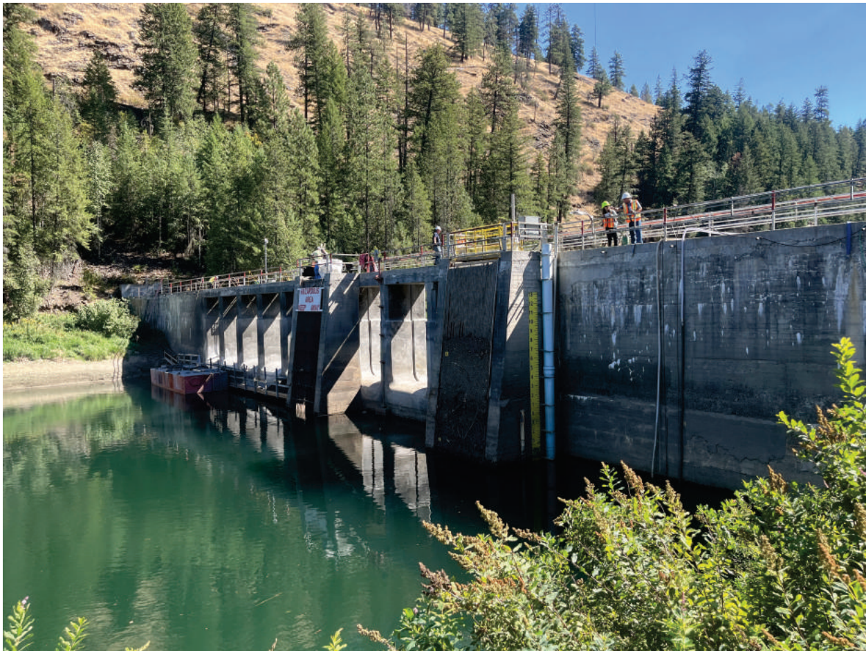
Figure 4.3-2. Upstream face of the dam showing intake structure.
